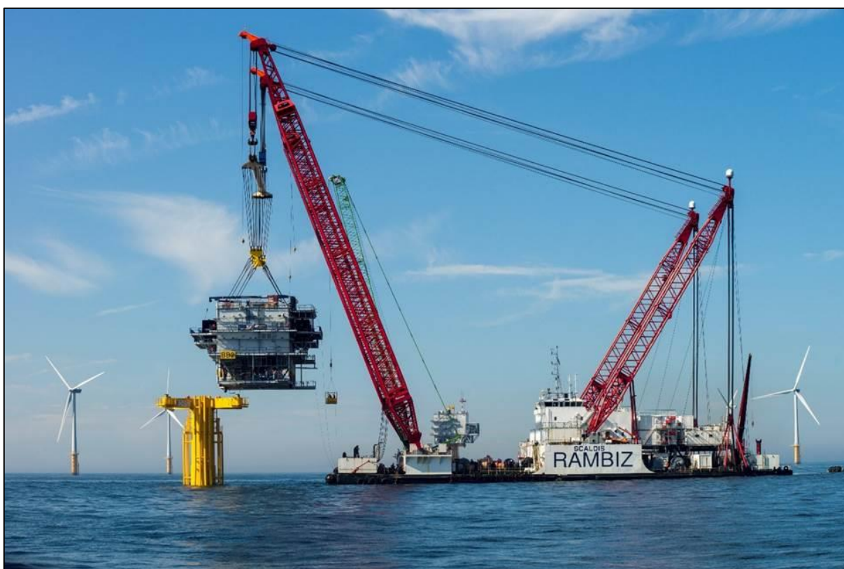
Figure 5-10: Heavy Lift Vessel installing an OSS Topside.
