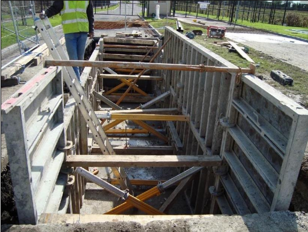
Figure 5-18 Photo showing joint bay under construction (in-situ).
