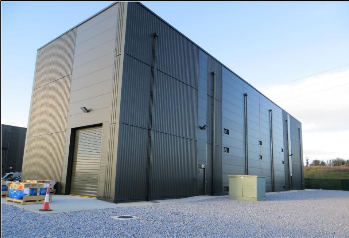
Figure 5-28: Photo of 220 kV GIS Substation Building.
