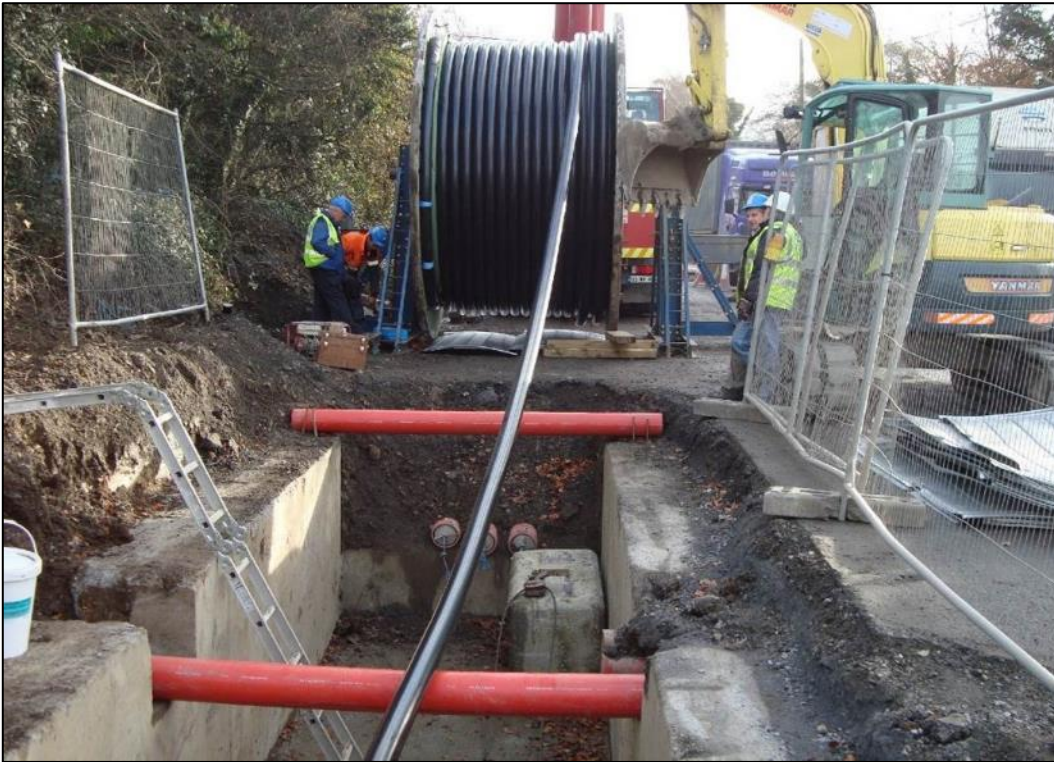
Figure 5-20 Photo of cable pulling procedure.
