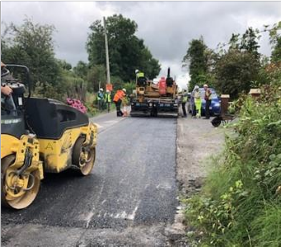
Figure 5-22: Permanent reinstatement of road surface over trench.
