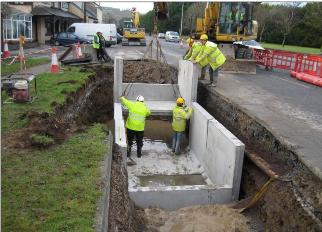
Figure 5-19 Photo showing joint bay under construction (pre-cast)
