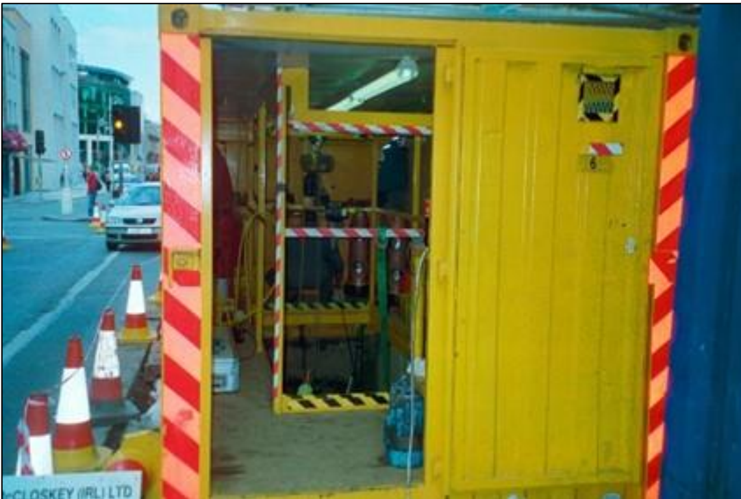
Figure 5-21: Photo of jointing container.
