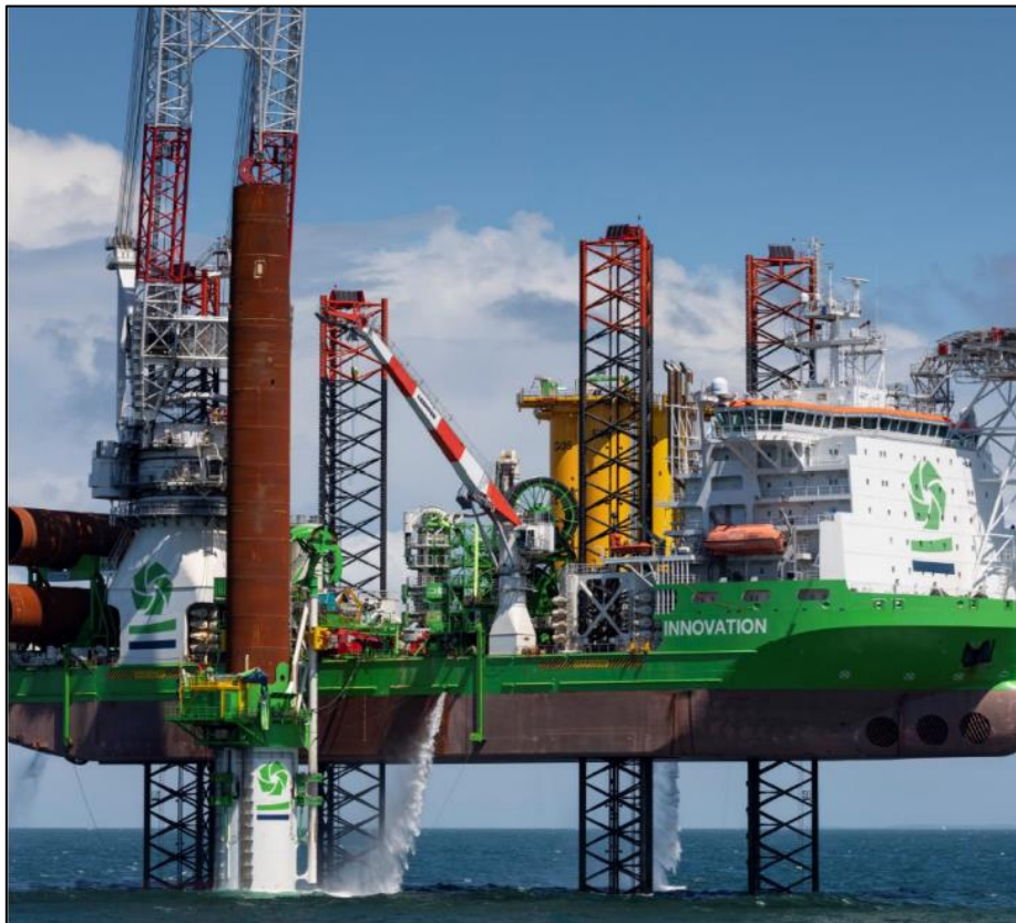
Figure 5-8: Monopile foundation installation from a JUV.
